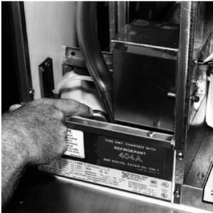
After turning ON the fresh water supply, check the connections on top of the Maximicer and all other connections for leaks. Check the water supply to the sump inside the ice machine by depressing the float valve or by activating the solenoid water valve. If you encounter any leaks or problems refer to the **Troubleshooting** section.
