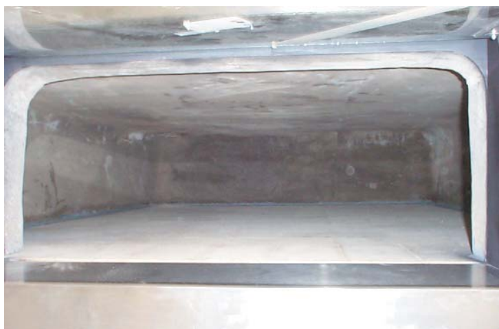
Inside the oven. This particular oven is 2.5m x 3m OD
