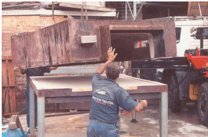
Oven arrives in 2 or more pieces and assembled on site
